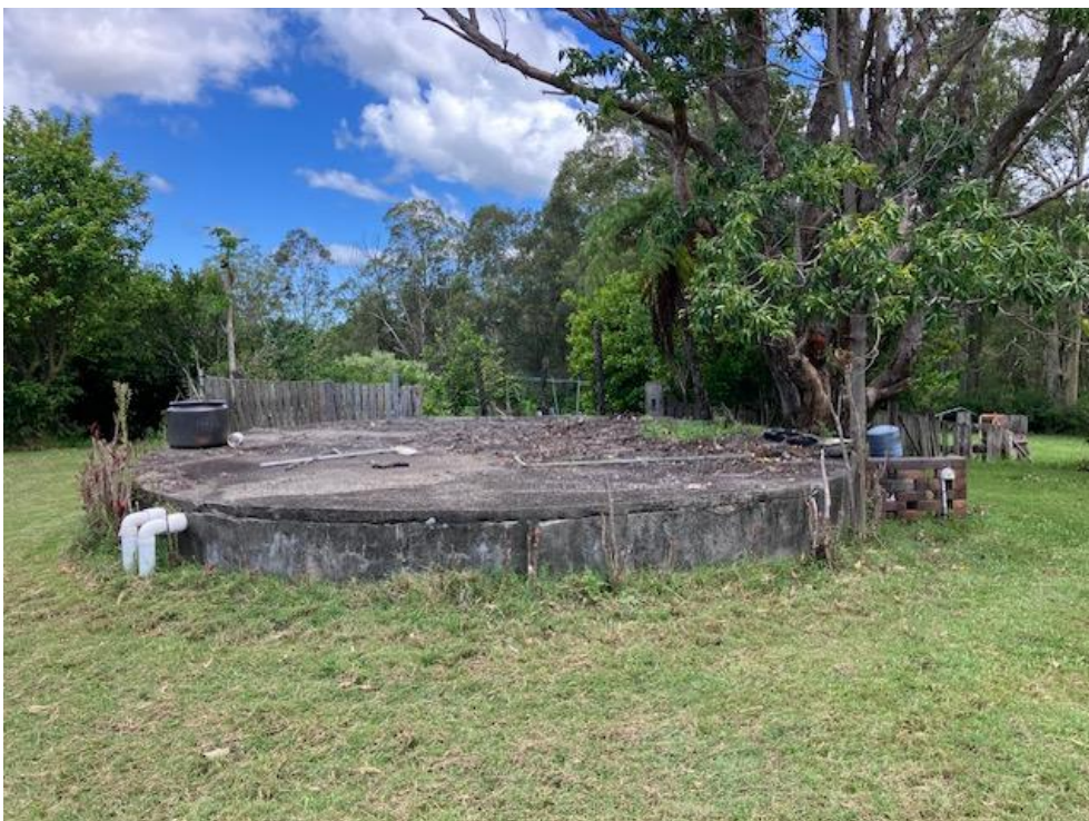
Existing inground concrete rainwater tanks servicing the existing dwelling which will be located on proposed Lot 105
